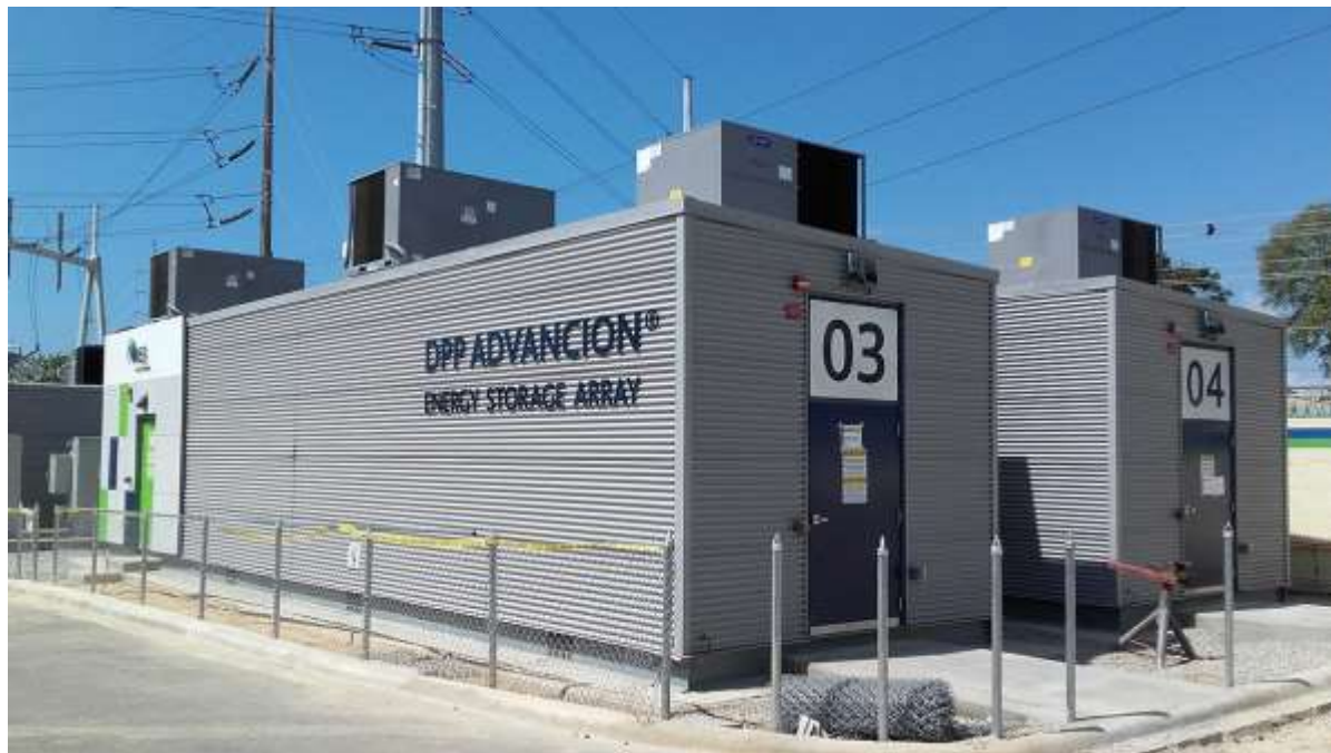
Santo Domingo, Dominican Republic 10 MW / 10 MWh, Frequency Regulation/Control Alternative to generators
