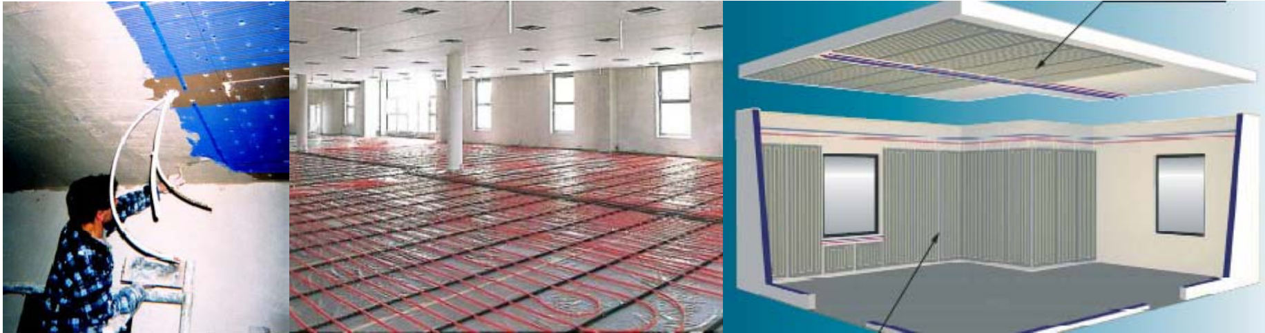
Low temperature radiant terminals
