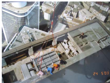
Extension + exchange of refrigerating machines
